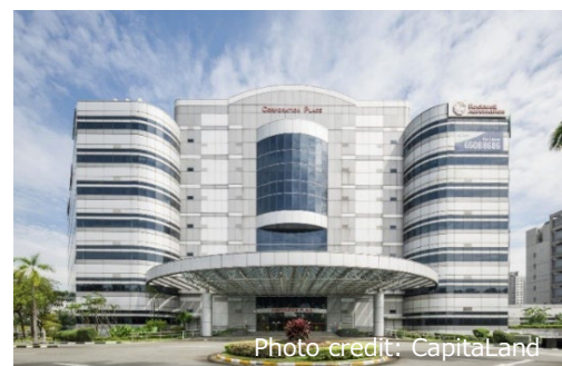
<An overall view of Corporation Place >
