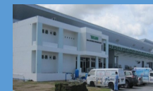
KAGA ELECTRONICS (THAILAND)
