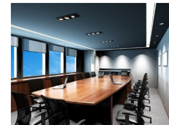
LED照明無線制御
