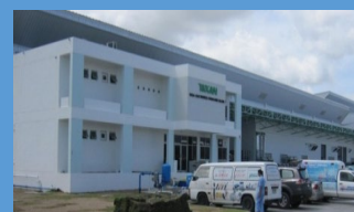
KAGA ELECTRONICS (THAILAND)
