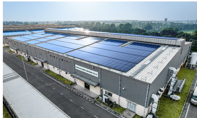
Solar panels installed at Vietnam factory
