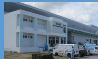
KAGA ELECTRONICS (THAILAND)
