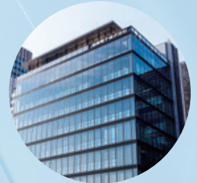
Kaga Electronics Head Office
