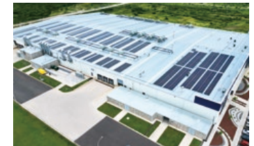
TAXAN MEXICO's New Plant
